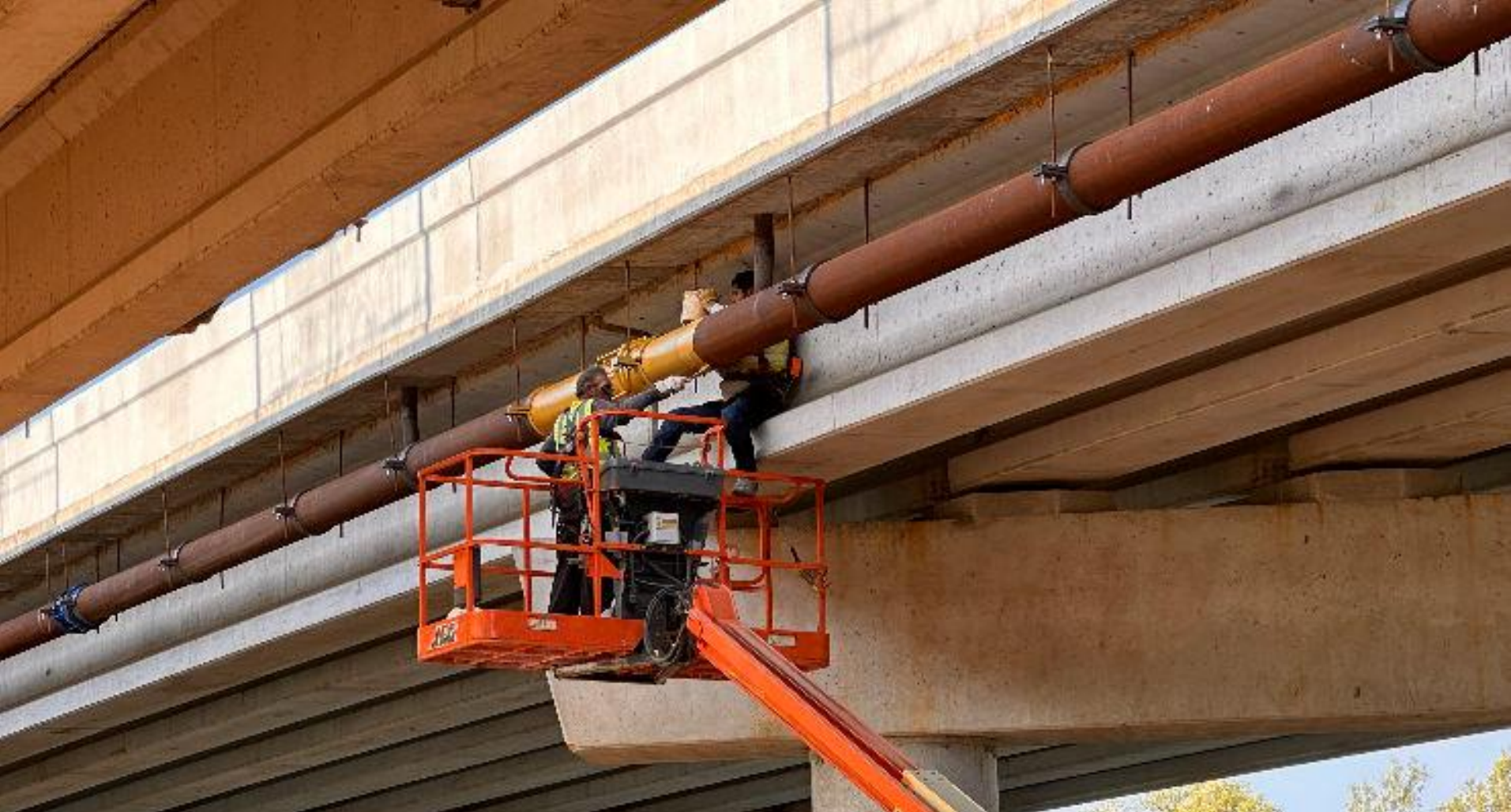
09-02-2026 – the contractor continued applying the approved coating to the bridge drain system underneath Units 28 and 29.
