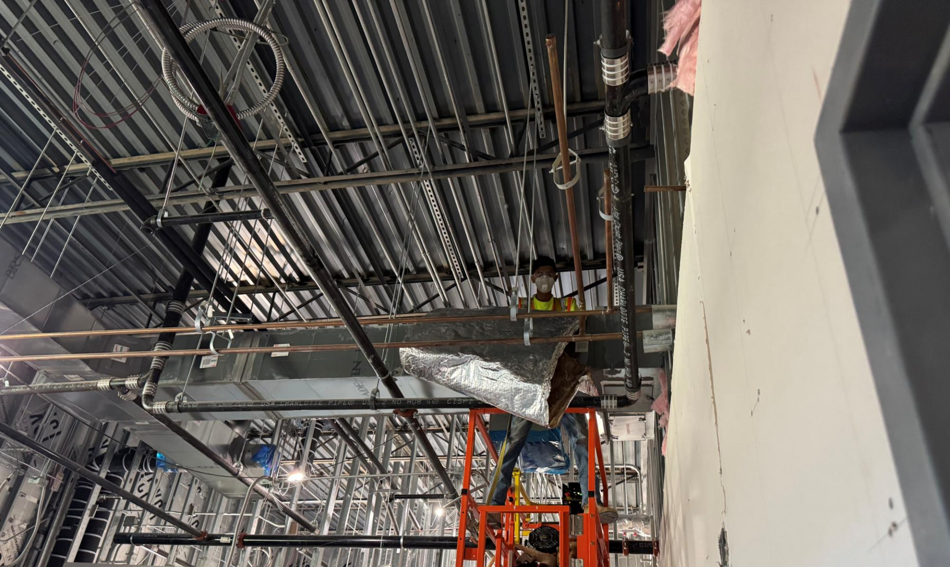
08-27-2026 – the contractor continued installing insulation around the ductwork for the air-conditioning system at the Agricultural Building.
