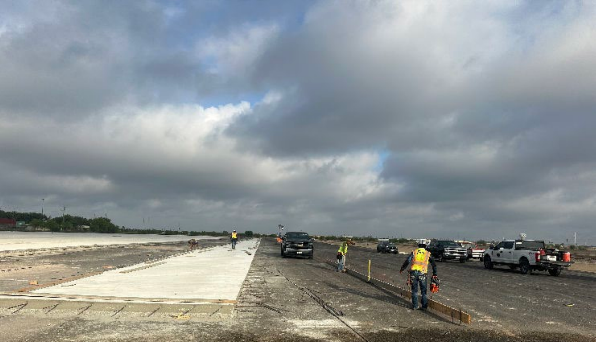
07-30-2026 – the contractor installed wood form to establish a new 15-foot by 730-foot concrete pavement section, beginning at the south parking lot pavement edge and extending approximately 245 linear feet north.
