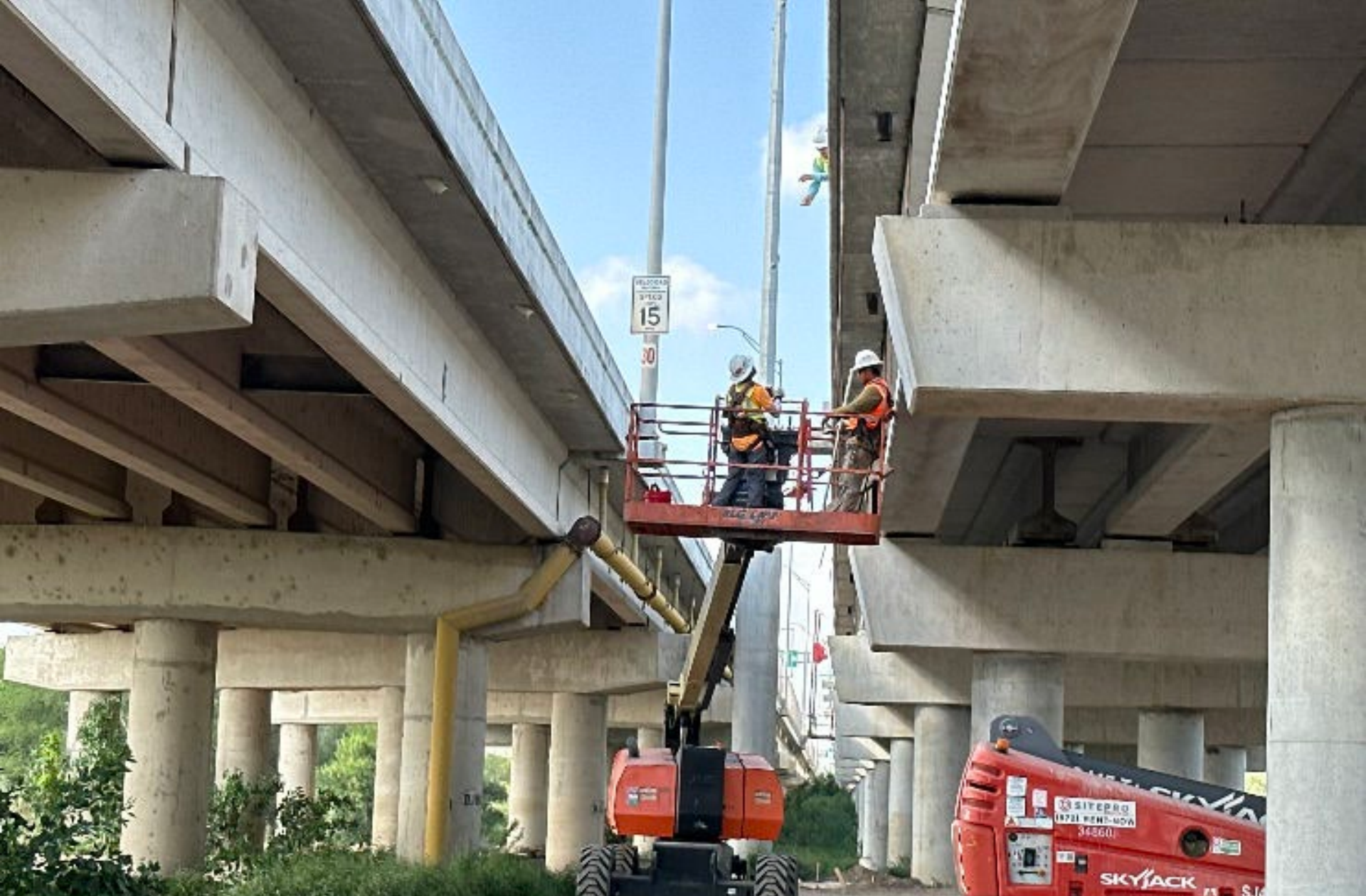
07-30-2026 – the contractor continued work on the bridge drainage system that runs beneath Unit 28 and 29.
