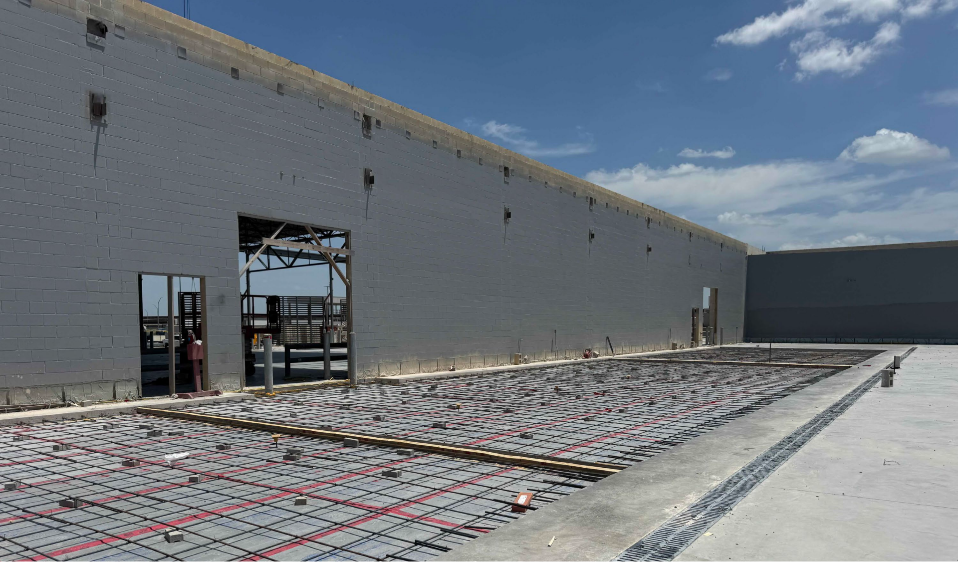
07-30-2026 –the contractor began installing wood formwork for the keyway as part of the repair work at the Cold Storage Building.
