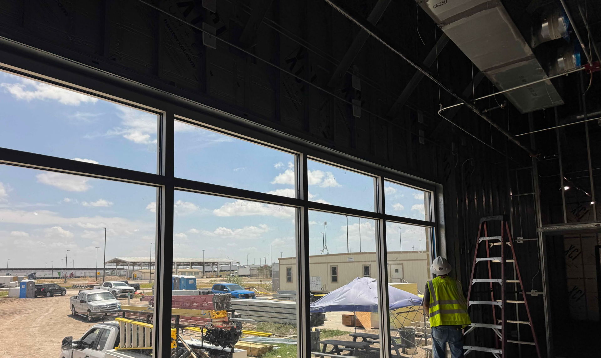
07-30-2026 – the contractor continued sealing the windows on the north and south side of the Agricultural Building.
