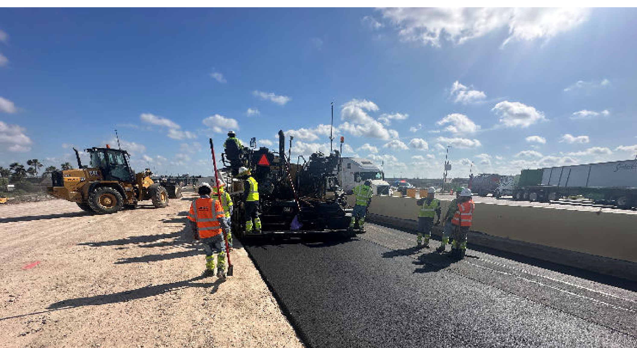
07-03-2026 – the contractor performed hot mix asphalt paving operations within the new roadway
