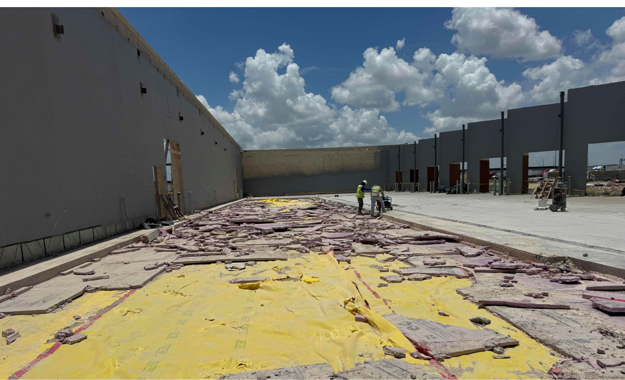
07-06-2026 – the contractor continued saw-cutting and removing concrete slab located along the east side of the Cold Storage Building.
