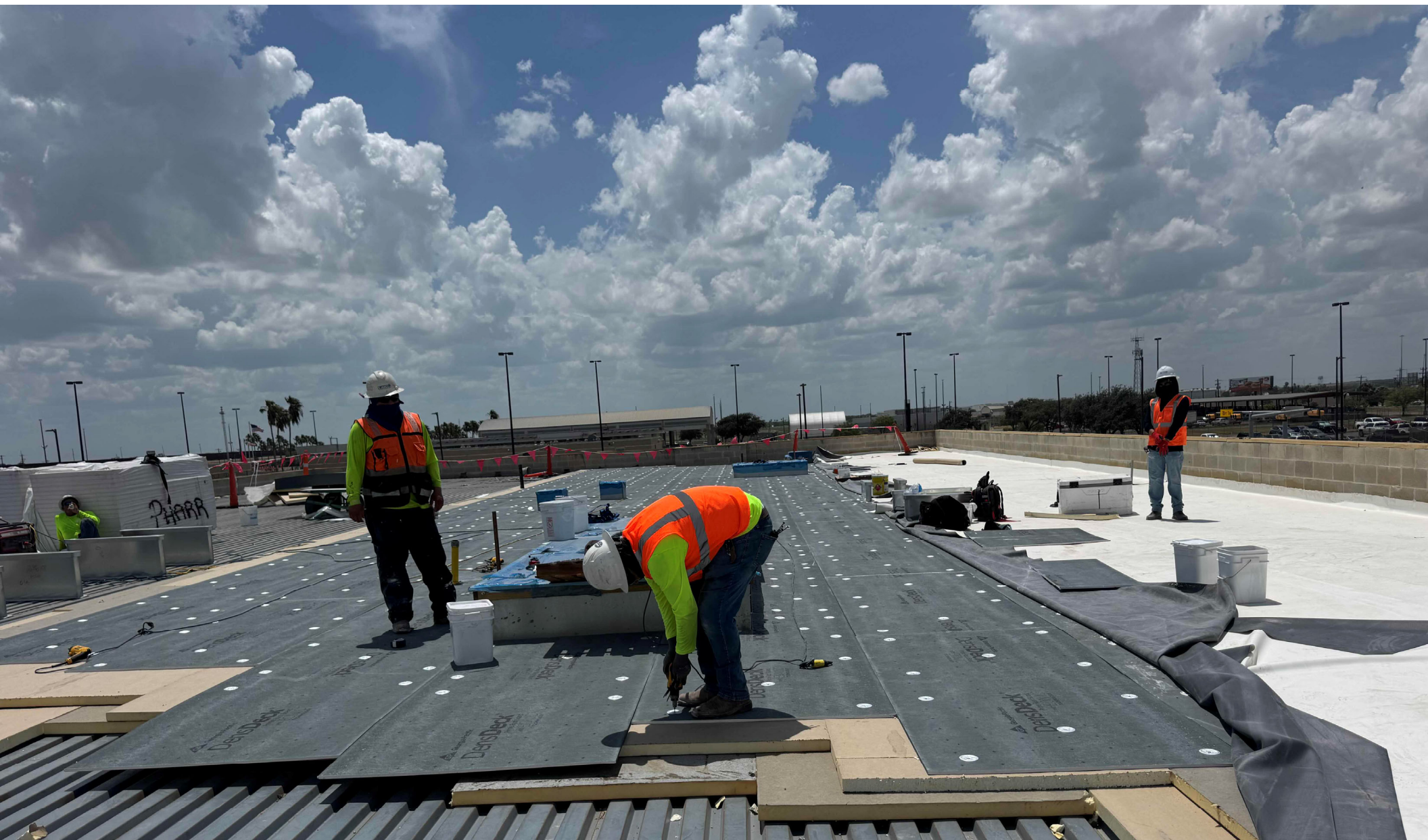
07-06-2026 – the contractor continued the of the roofing system assembly, including the 6-inch rigid roof insulation, ½-inch glass mat reinforced gypsum cover board, and EPDM roofing membrane, on the roof of the Agricultural Building.
