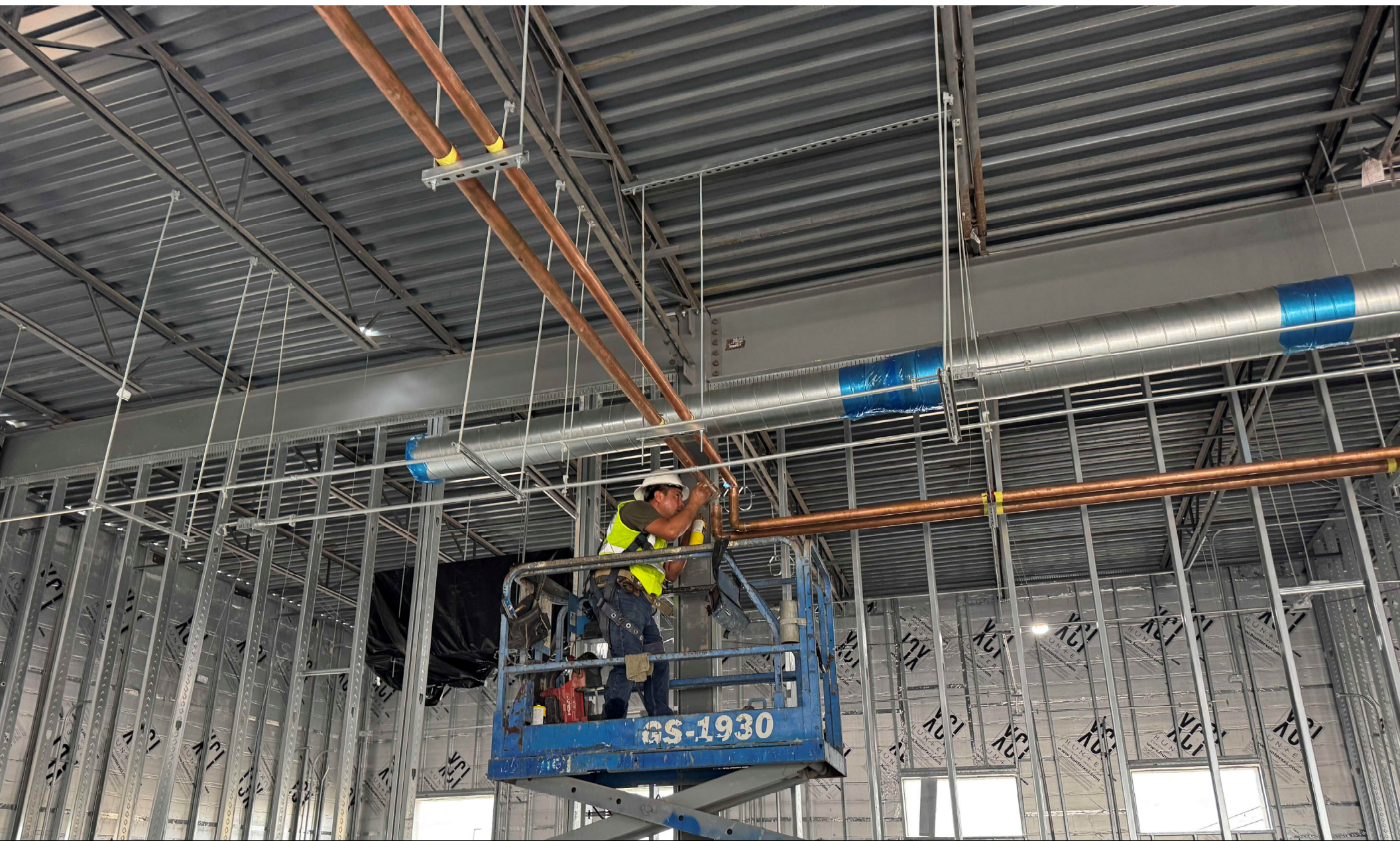
05-07-2026 – the contractor continued installation of ceiling hangers for the domestic water piping at the Agricultural Building.
