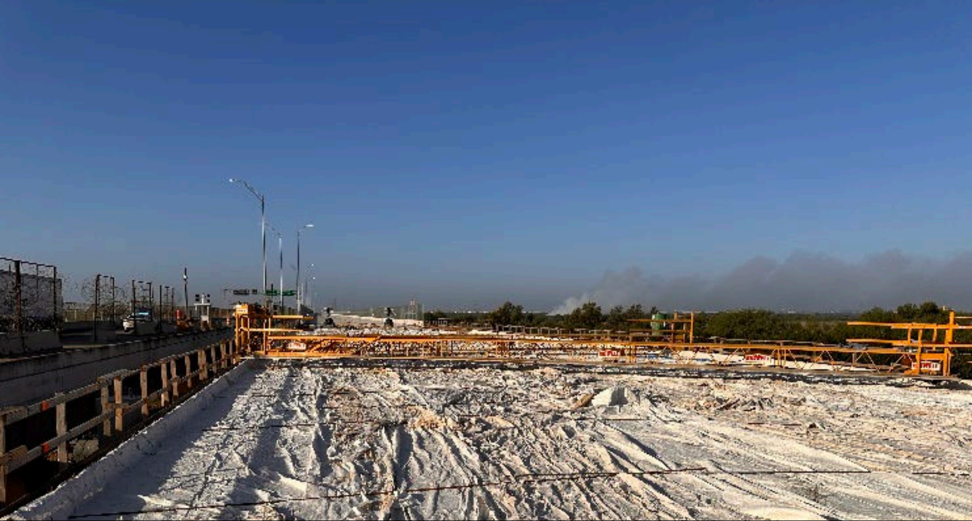
05-13-2026 – the contractor completed a concrete pour overnight at unit 29 (the unit connecting to MX) and then laid out curing blankets over the concrete surface to assist with moisture retention and promote proper curing conditions.
