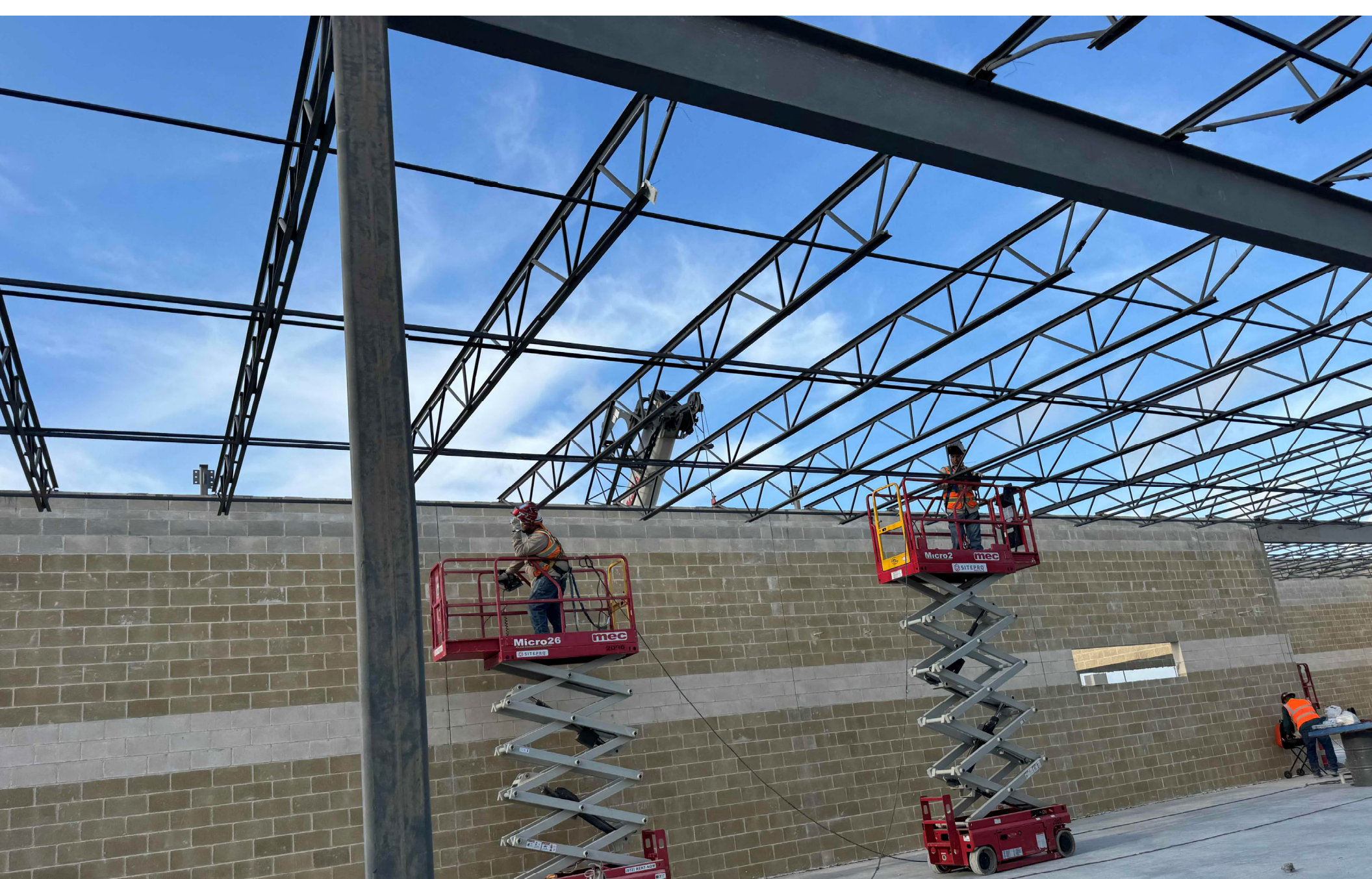
04-02-2026 – the contractor continued installing steel bridging for the steel joist in the Agricultural Building.
