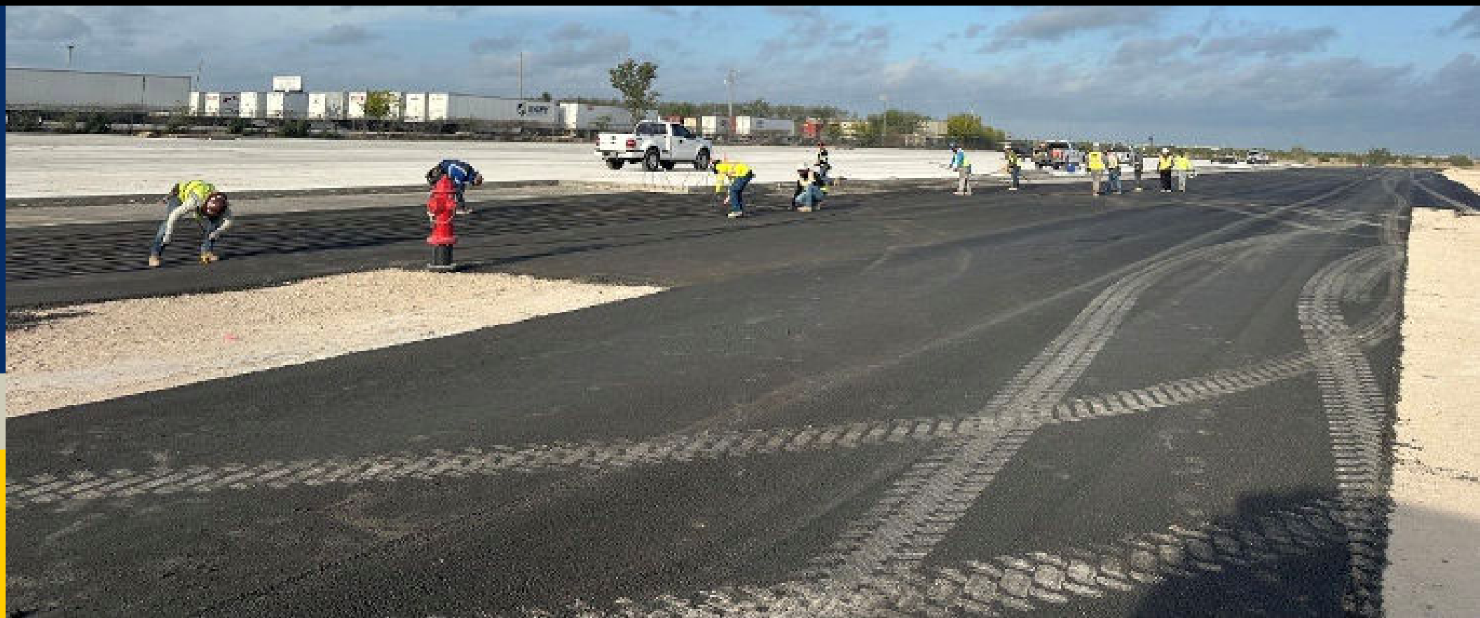
04-02-2026 – the contractor installed reinforcing steel (#4 and #5) in Section 5 and 6 in accordance with project plans.
