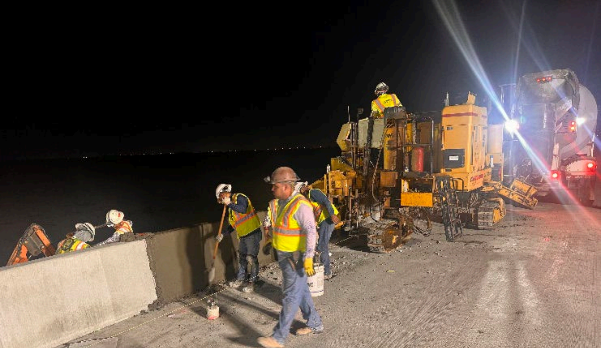
03-25-2026 – the contractor continued with the concrete pour for the single-slope traffic rail, progressing with placement in accordance with the project plans.
