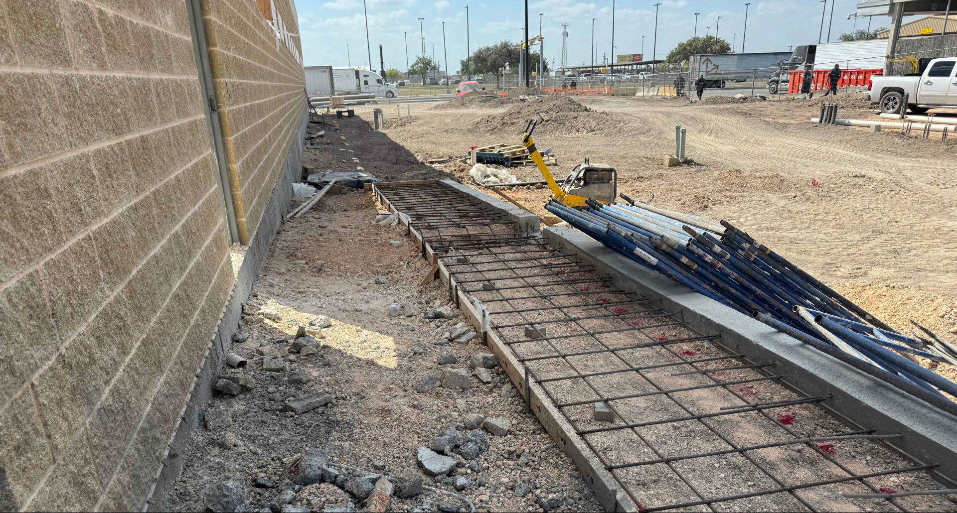
03-30-2026 – the contractor began installation of concrete reinforcement for the walk-up ramps located on the north and west side of the Agricultural Building
