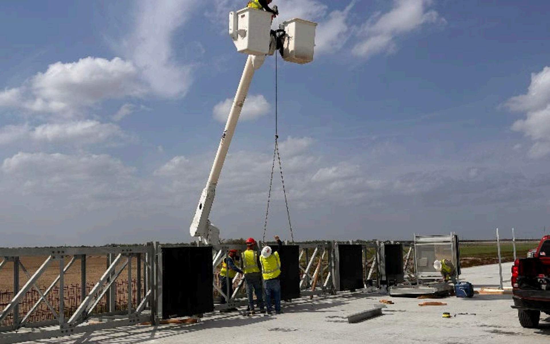
03-09-2026 – D&G's crew began installing the full-color LED DMS assembly (5' x 5') on the HOSB structure located on the bridge slab at Unit 36.
