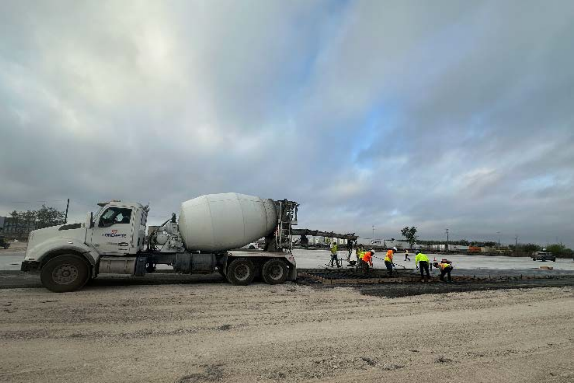
03-05-2026 – The Maverick Company crew placed 7.5-inch Continuous Reinforced Concrete Pavement in Sections 3 and 4. Operations included concrete delivery, placement, consolidation, finishing, and general housekeeping activities.
