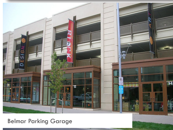
Parking Garage with first floor retail
