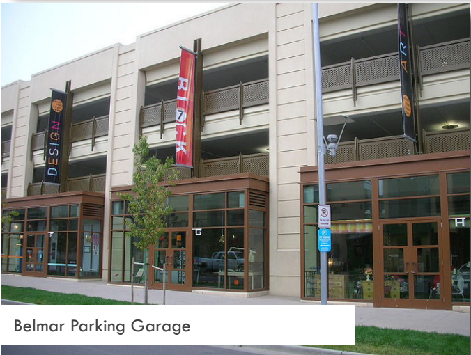
Parking Garage with first floor retail
