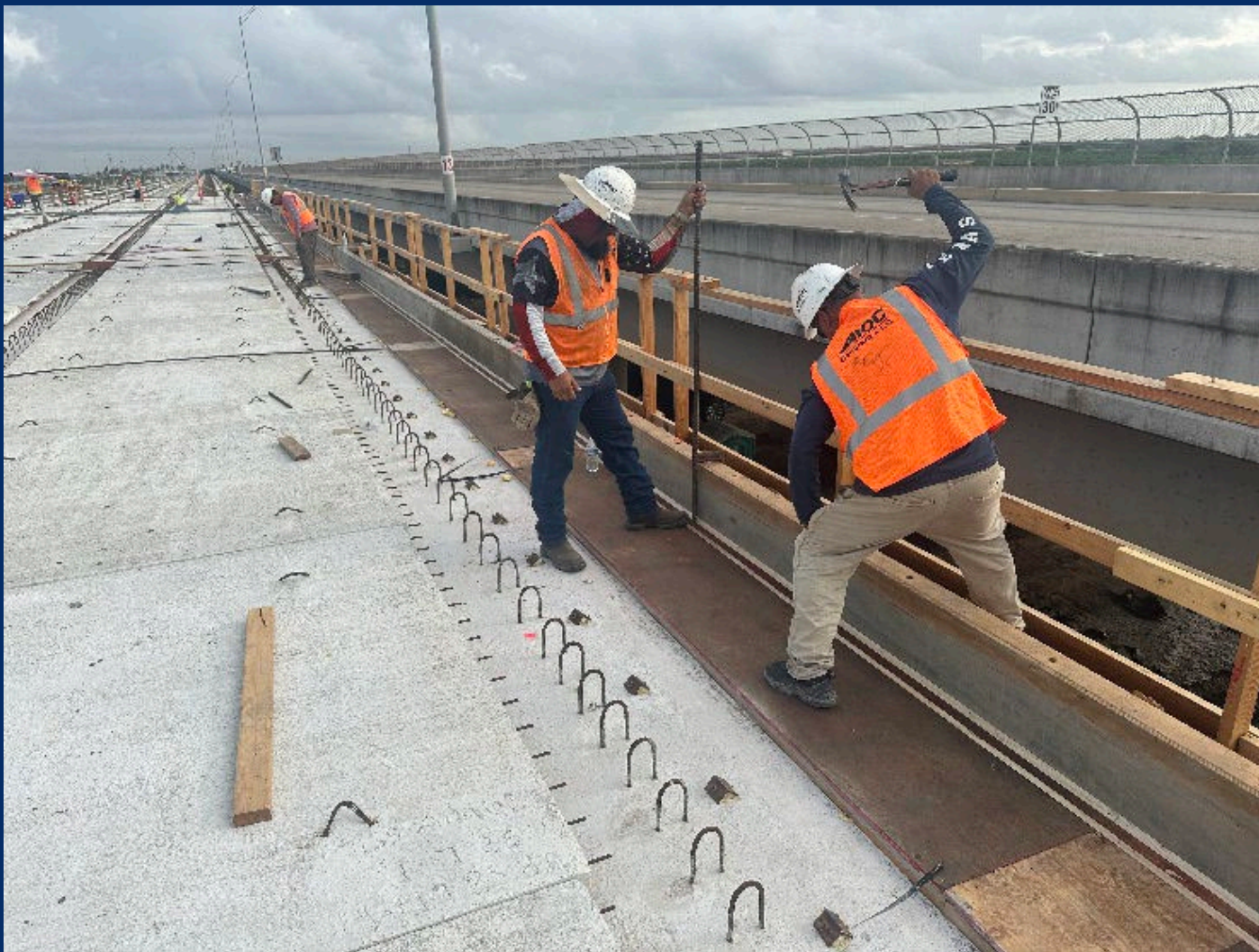
10-14-2025 – Crew installing wood form railings at the east and west ends of Unit 42.
