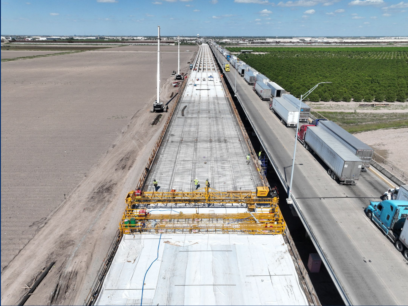
10-15-2025 – Around Unit 42 looking north.
