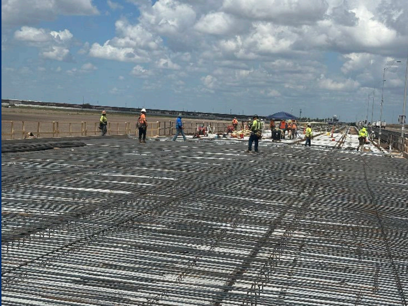
09-24-2025 – Crew continued tying bridge deck steel rebar at Unit 39.
