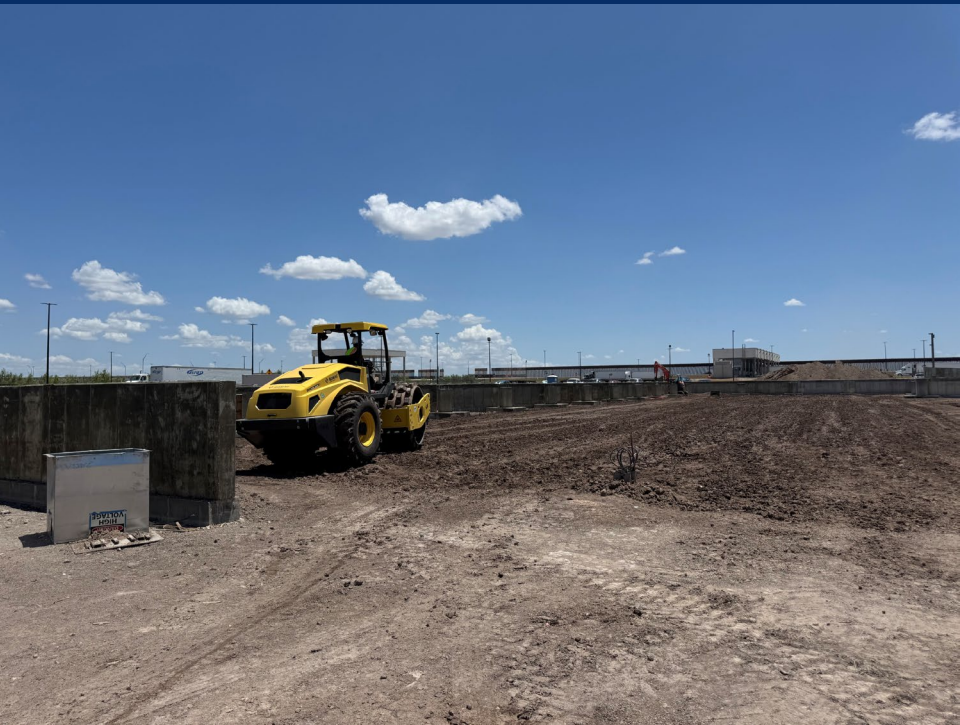
08-12-2025 – Contractor continued grading and compacting the subgrade for the dock expansion.
