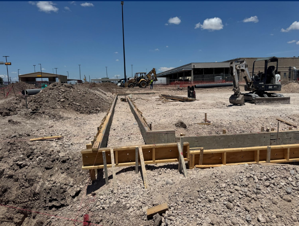
08-12-2025 – Contractor continued installing wood formwork for the footings of the Agriculture Lab building.
