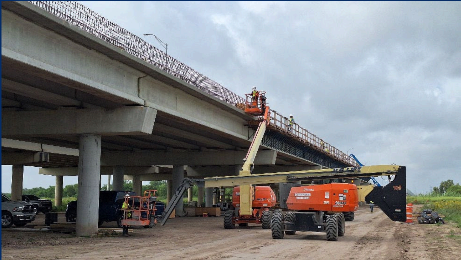
07-15-2025 – Crews continue installing the overhang forms and railing.
