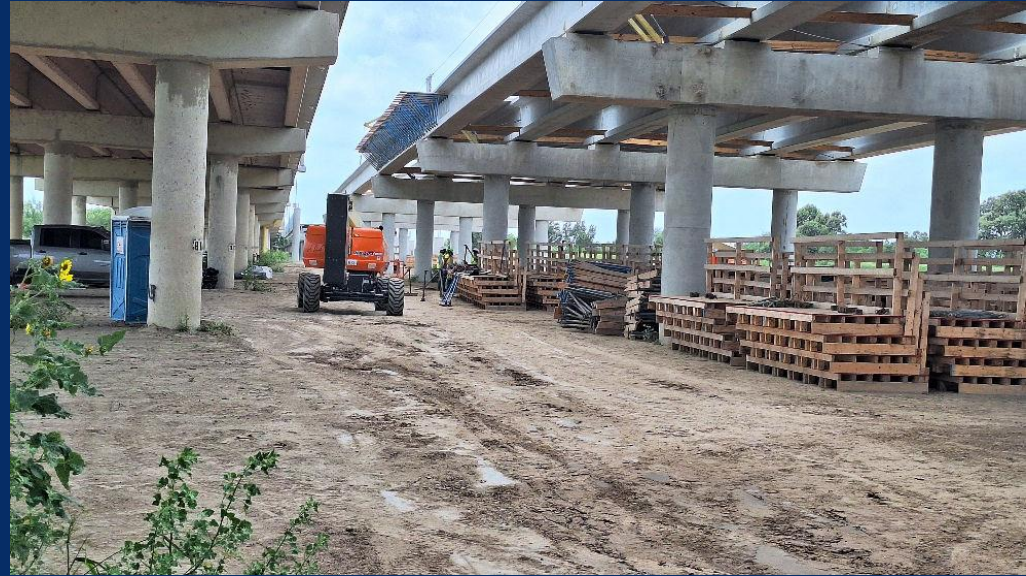
05/23/2025 – Installation of bedding strips and the overhand brackets.
