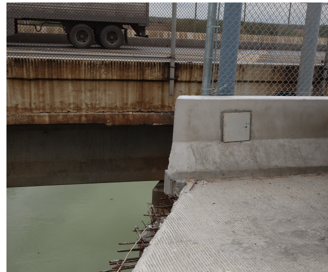
EXISTING CONDITION AT BENT 104 JOINT
