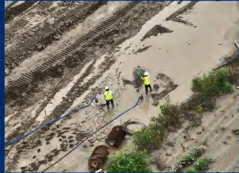
March 31, 2025 – Laborers dewatering the ROW.
