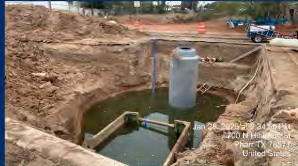
January 28, 2025 – Manhole on W. Sioux Rd.
