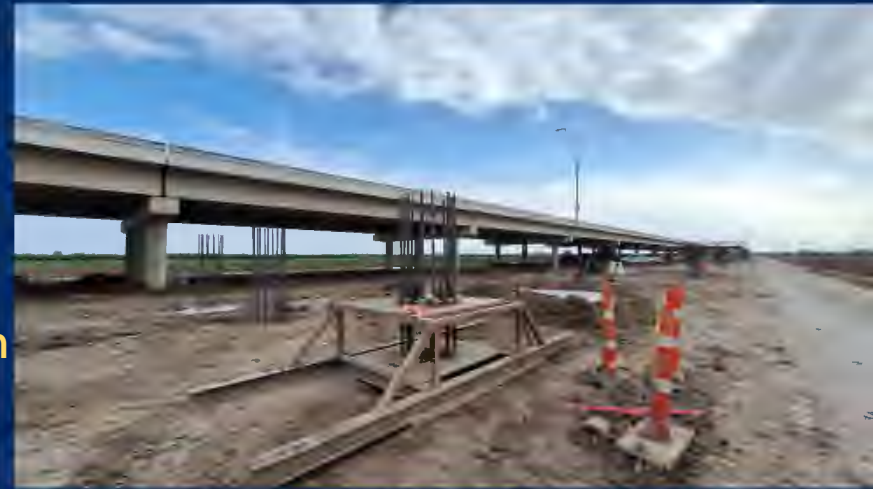
January 30, 2025 – The dowels placed in the 60” drilled shaft foundations at Bent 149-152.
