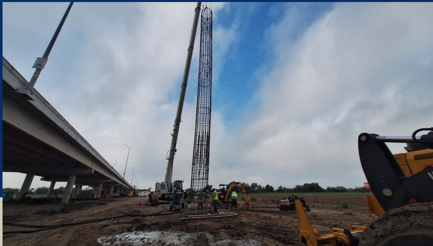
Daily Activity Report 9-18-2024 – Drilling rig was used to drill 69 LF for the (middle) 60 IN drilled shaft foundation at Bent 114.
