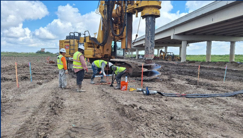
Daily Activity Report 9-18-2024 – Drilling rig was used to drill 69 LF for the (middle) 60 IN drilled shaft foundation at Bent 114.
