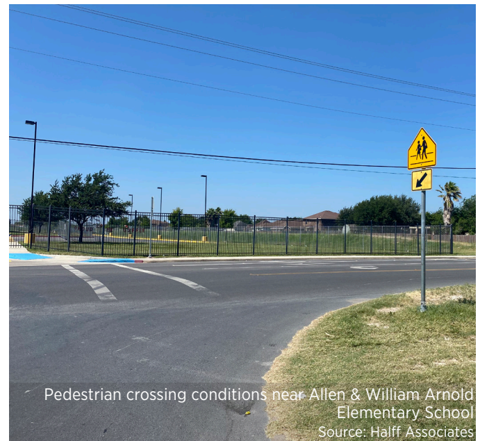
Students walk to LBJ Middle School in the grass due to a lack of sidewalk infrastructure Source: Halff Associates
