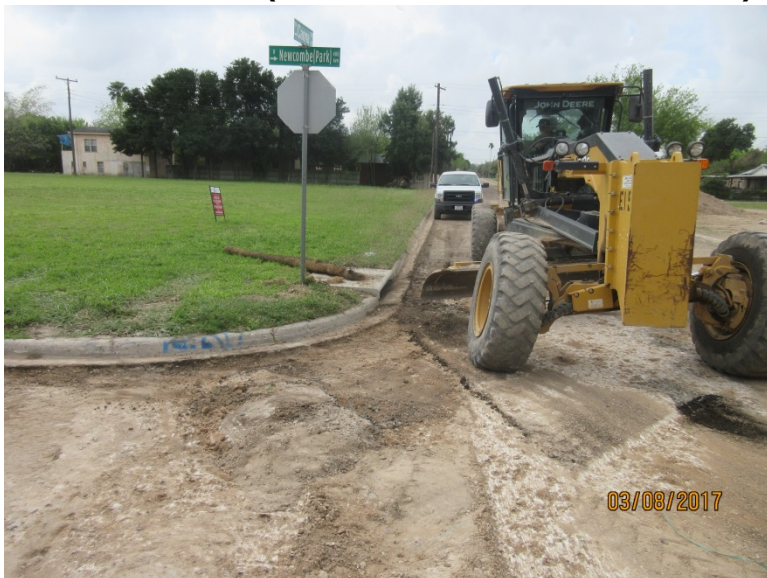
Water Line Transmission Improvements (Prepping Road)
