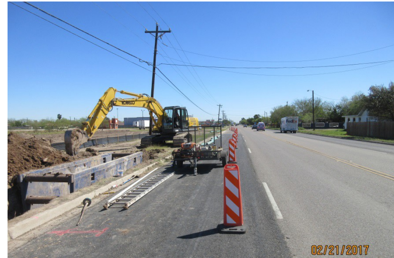
South Pharr Development and Research Center Off Site Utilities
