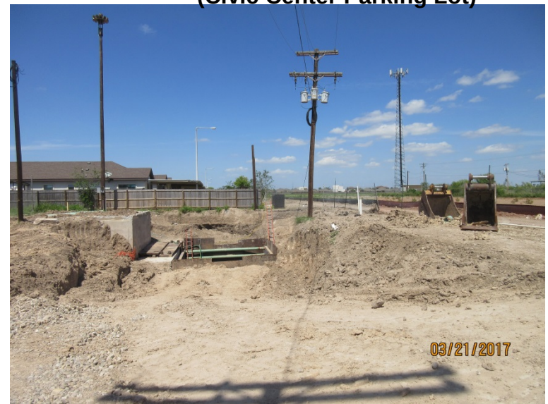
Lift Station #25 and Force Main (Excavation for New Lift Station No. 25)
