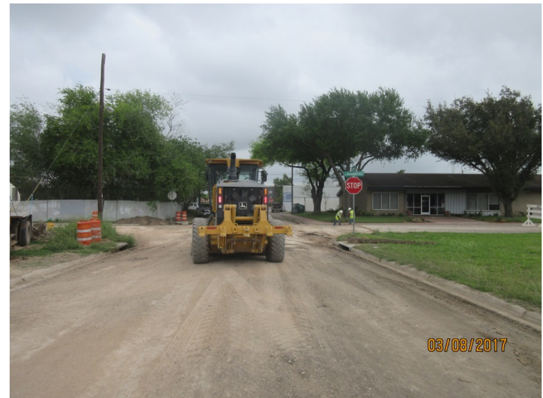
Water Line Transmission Improvements (Prepping Road)
