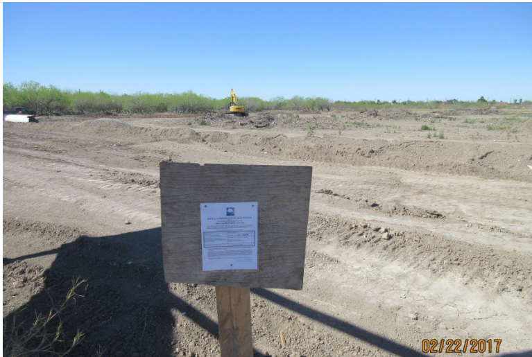
South Pharr Development and Research Center Off Site Utilities (Small Construction Site Notice)
