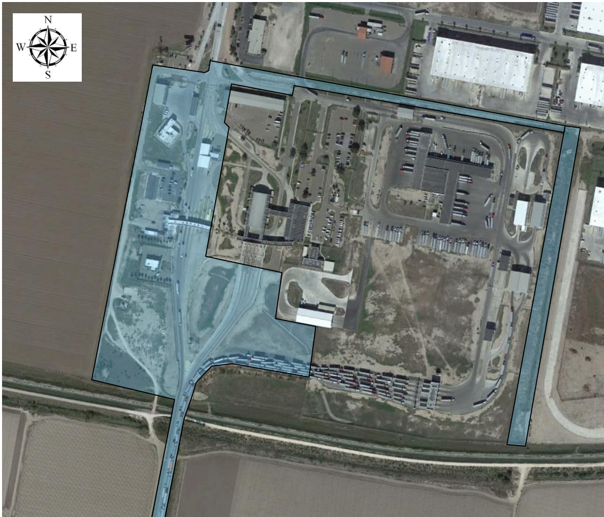
Figure 2: Aerial view of the Pharr International Bridge. Areas highlighted in blue are to be evaluated as part of this scope of work for the Maintenance Plan.
