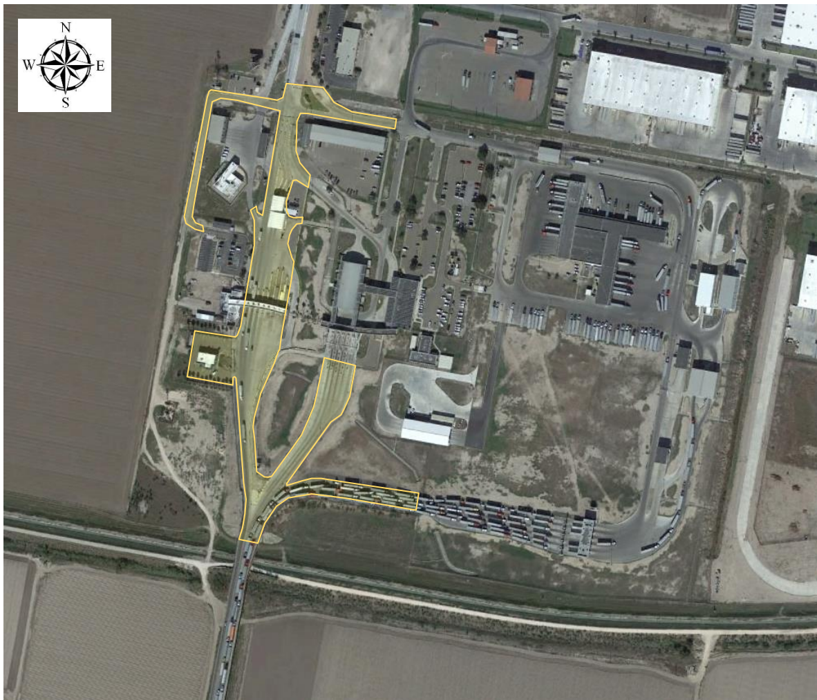
Figure 1: Aerial view of the Pharr International Bridge. Areas highlighted in yellow are to be evaluated as part of this scope of work for the Pavement Assessment.
