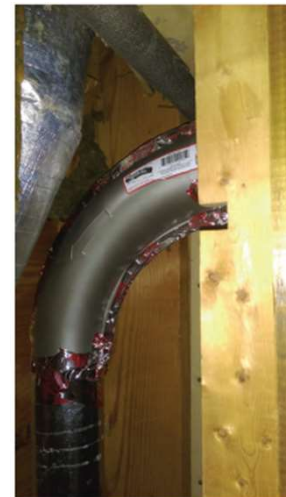
Joints in dryer exhaust duct must be sealed.
