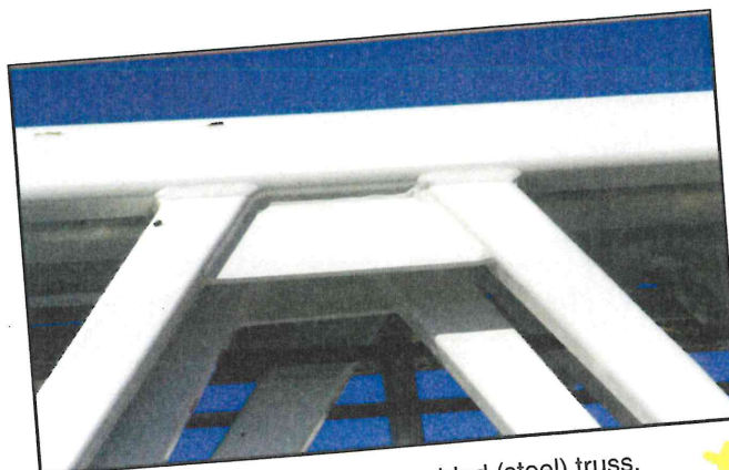
Figure 16.6a An example of a welded (steel) truss.
