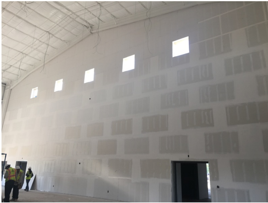
Image 5. Taping and floating installation completed.
