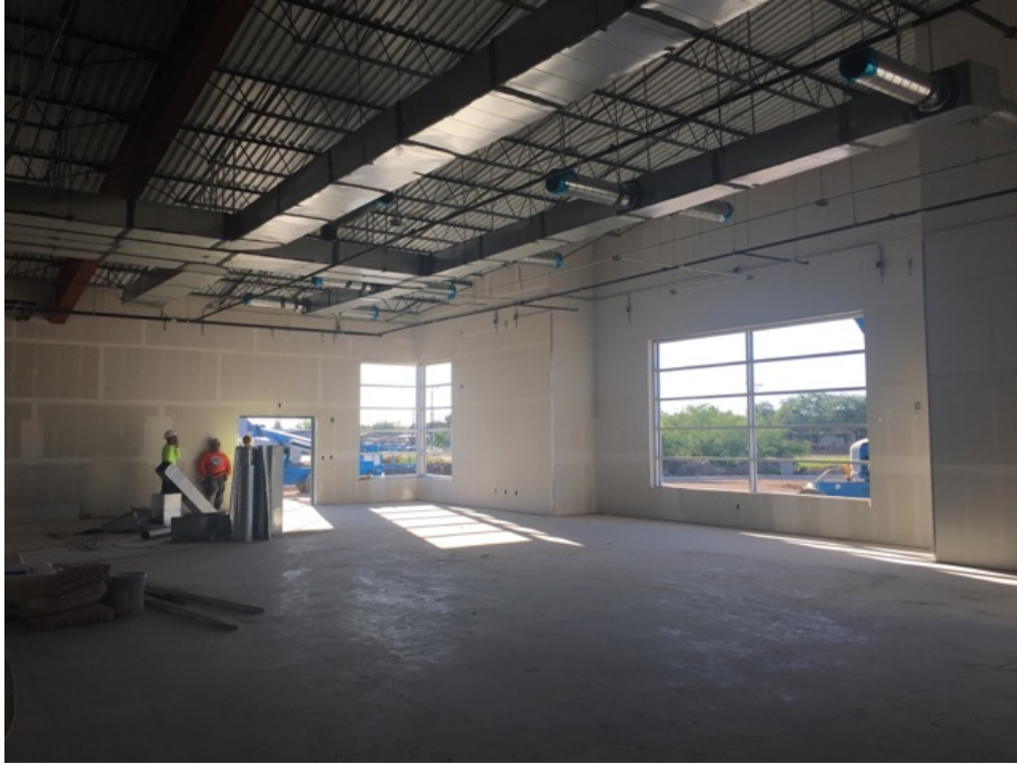
Image 4. Window frames installation complete.
