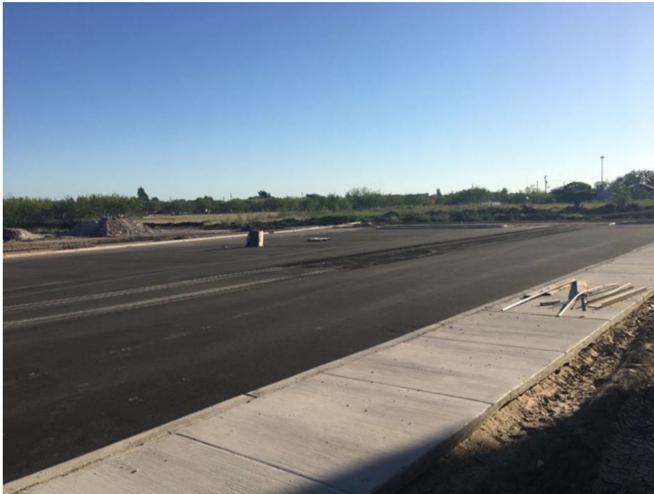
Image 7. HMA north parking lot. 85% completion.
