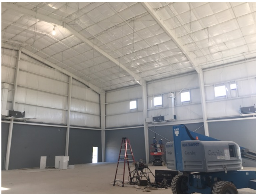
Image 6. A/C ventilation ducts installation in progress.
