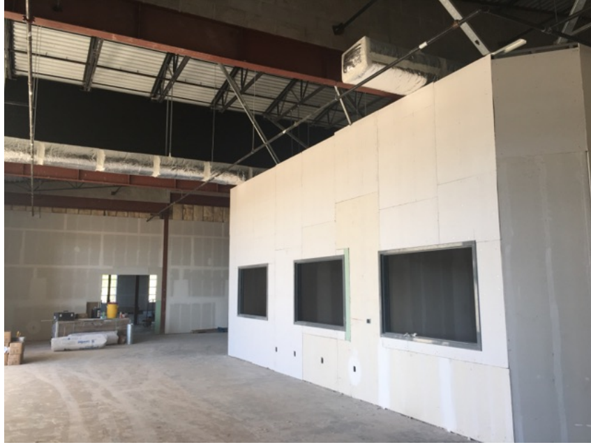
Image 2. Gypsum wallboard and insulation installation in progress.
