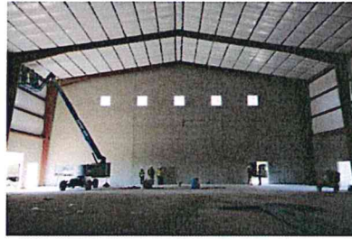
3.8 Exhibit Hall structure has been completed, pending windows.
