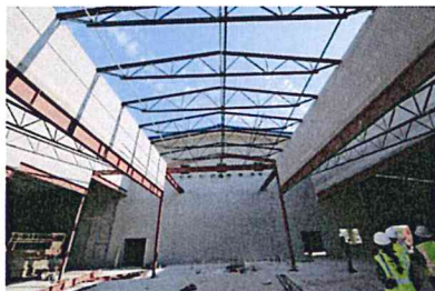
3.5 Masonry work and steel erection is ongoing.
