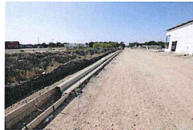
3.12 Concrete curb is ongoing on east side of the property.
