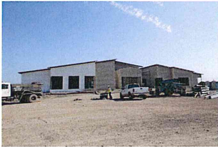
3.1 Over all building progress.
