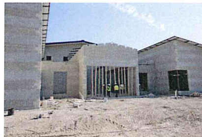
3.4 Masonry work and steel erection is ongoing.
