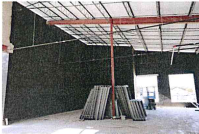
3.11 Waterproofing is ongoing.
