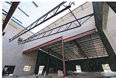
3.6 Steel erection has been substantially completed.
