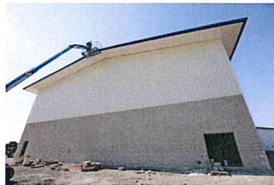
3.10 Soffit installation is ongoing.
