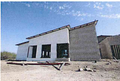
3.3 Paint primer is ongoing.
