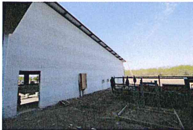
3.9 Bloc primer is ongoing.
