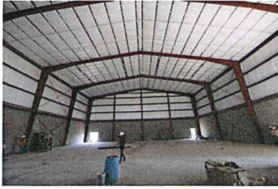
3.7 Exhibit Hall structure has been completed, pending windows.
