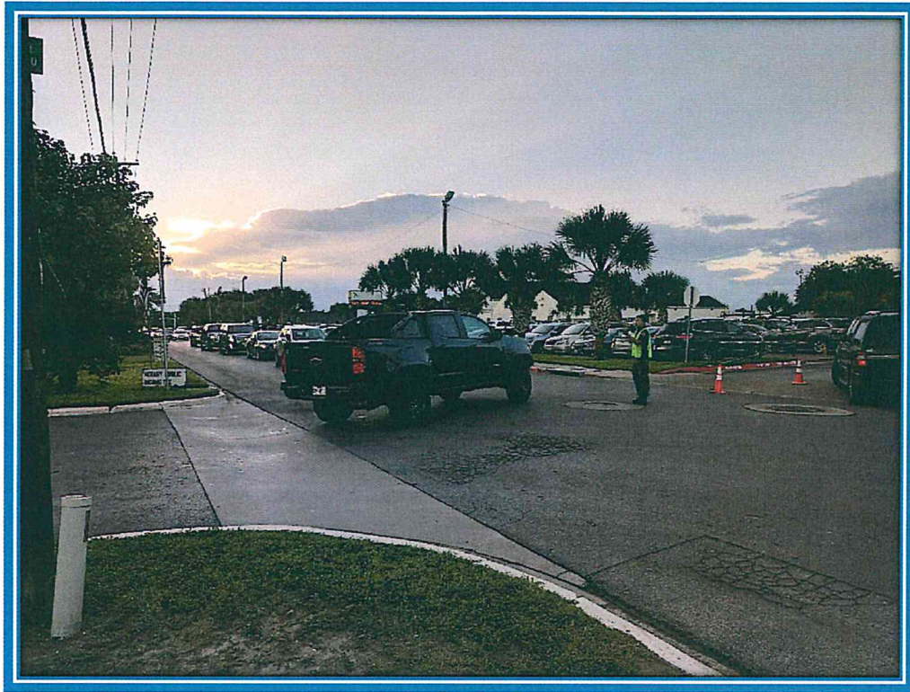
Facing East on Kelly Ave, to Project Site
