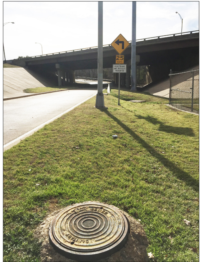
Carollo is performing a major water and wastewater main replacement for the City of Dallas that includes many complex site conditions.
