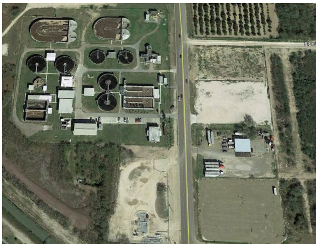
Aerial view of the City of Pharr's Wastewater Treatment Plant
