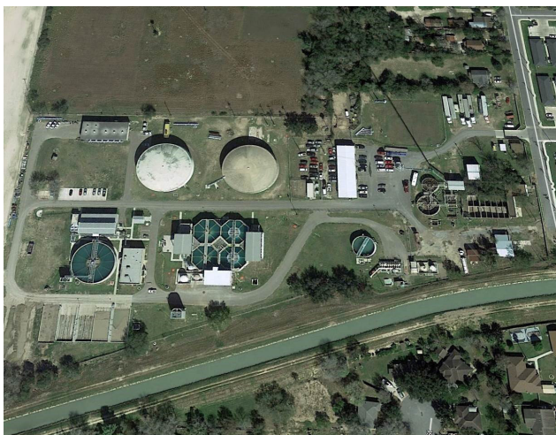
Aerial view of the City of Pharr's Water Treatment Plant
